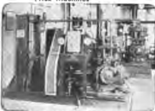
Two of the Eight Ammonia Refrigerating Units
