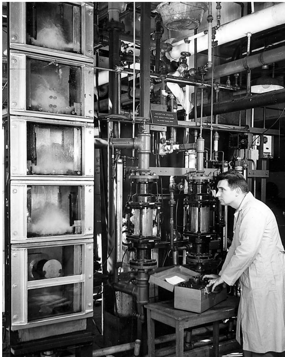
Larry Warzel (Ph.D. 1955, with Brymer Williams), using water to absorb carbon dioxide and other gases from an air stream in the investigation of tray efficiencies for a bubble-cap column. This project was the first in the country to be sponsored by the AIChE, and was located on the second floor of East Engineering, outside Room 2219.
