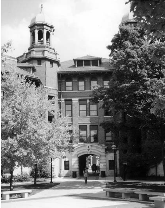
The “Engineering Arch” in the West Engineering Building (now renamed West Hall), taken from the northwest. July 2000.
