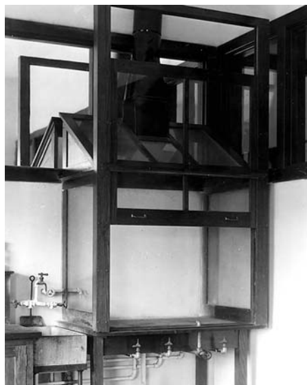
Original type of East Engineering fume hood.
