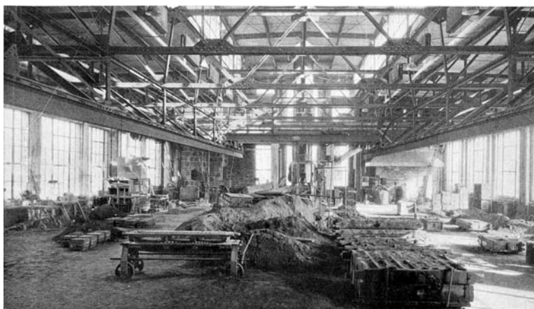
The main floor of the foundry is on the top floor, which allows a monitor roof and abundant light and air. It also prevents considerable nuisance in the neighborhood, since the fumes are discharged at a high level from the ground. The cupola is shown in the far end of the picture. A traveling crane traverses the whole length of the main bay.
